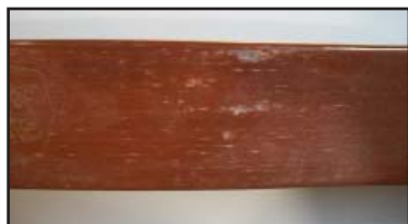
Figure 8: Indications of delamination.
